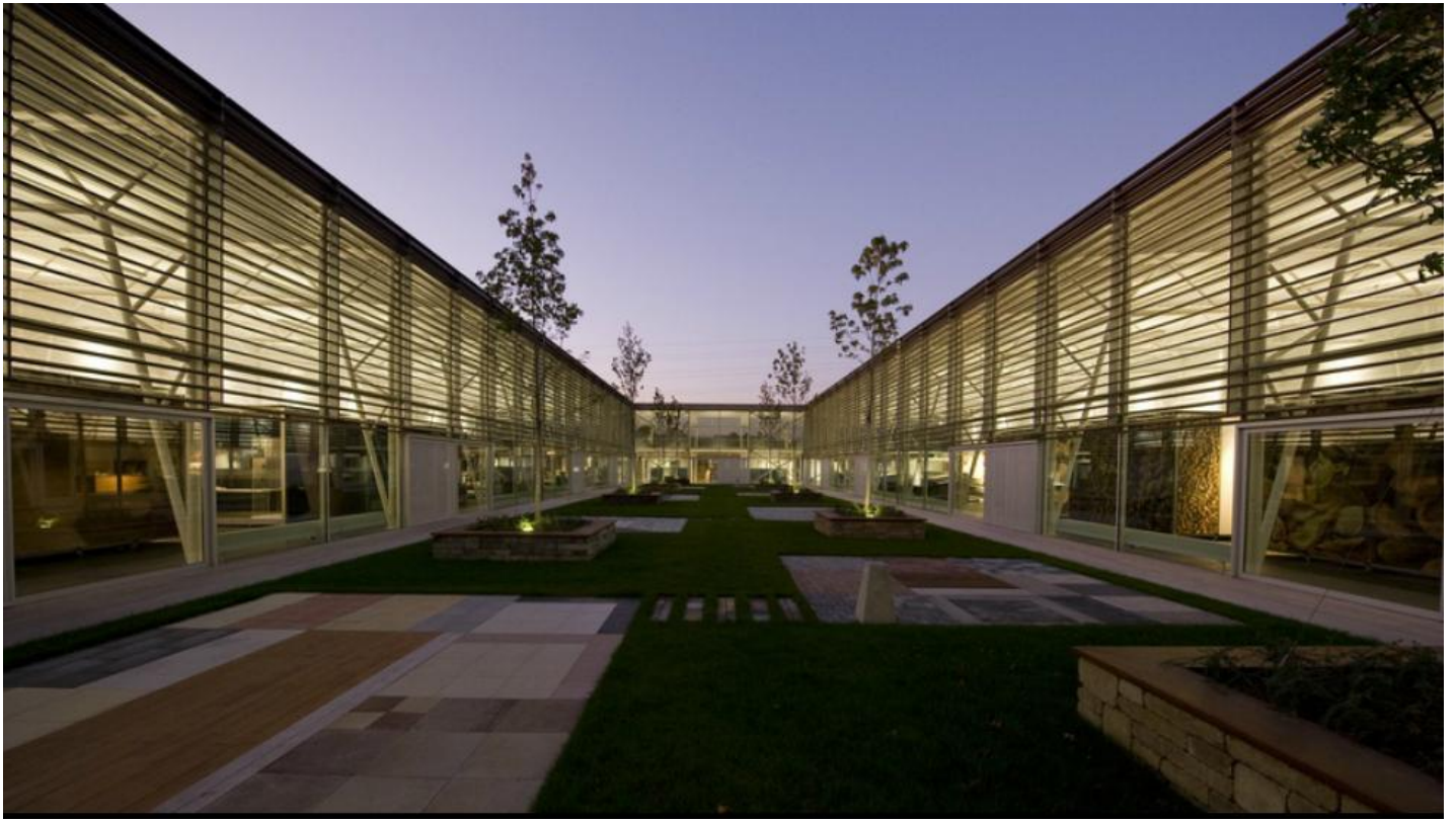
Getaz | Projekte von Saint-Gobain Building Glass | Saint-Gobain Building Glass
